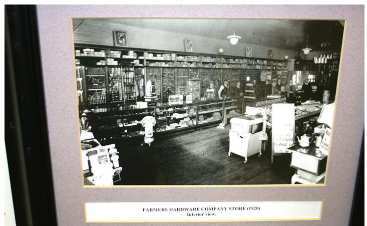
The old Farmers Hardware on Green Bay Street was razed to make room for the new Shawano Municipal Utilities structure. Radio Shack had most recently occupied the structure.
